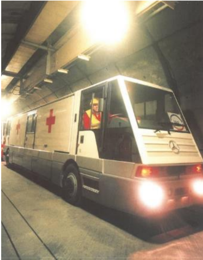
The service tunnel provides access to the tunnel for maintenance and rescue vehicles, among others. ( Link to high-resolution photo)
