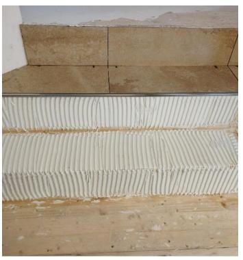
Due to the special stress on the stairs, the installation was carried out using the combined method. ( $\underline{LINK}$  to the photo)
