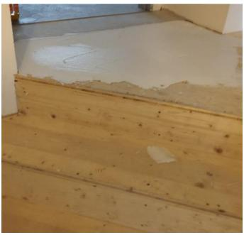
As PCI Flexcoll does not require priming, the adhesive can be applied directly after sanding and cleaning the substrate. (LINK to the photo)
